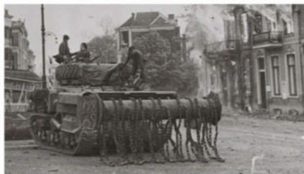
Sherman tanks were outfitted with flails to clear a path through minefields
